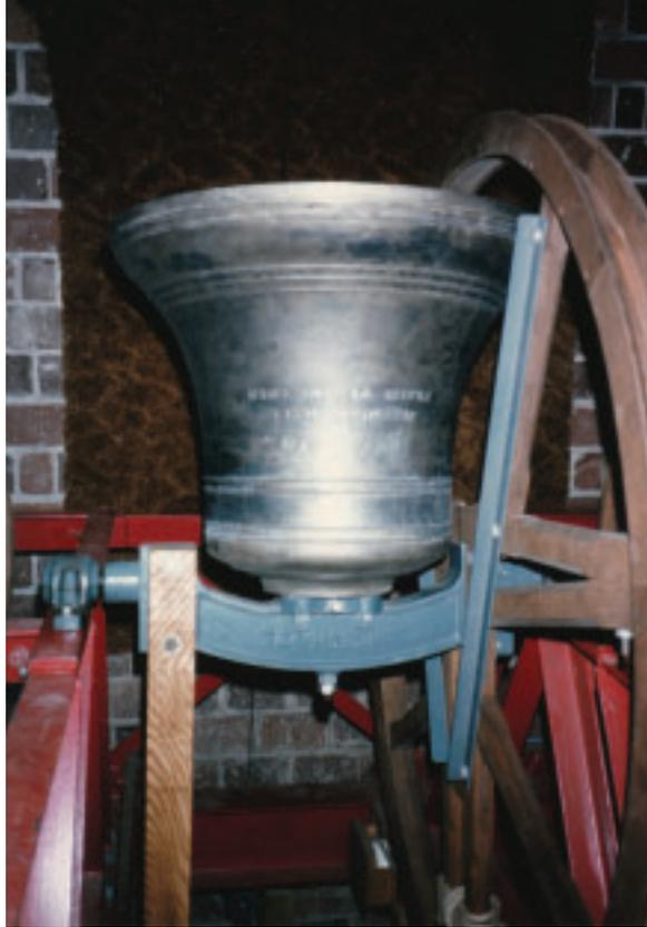
***This bell is "rung up" and ready for change ringing, where it will swing back and forth in a nearly 360-degree arc.***
